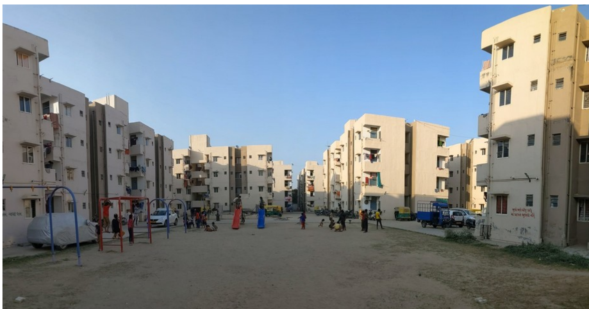
Figure 12: ARHC site with about 1,000 houses implemented and managed by a real-estate company near Thaltej, Ahmedabad; Source: Swastik Harish
