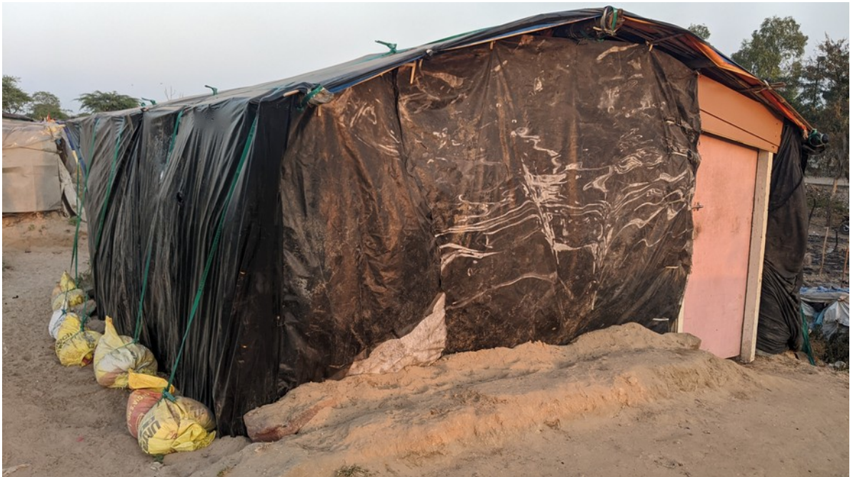
Figure 3: Construction technology of a typical house in most of the bastis visited, illustrating the kutcha nature of building materials; Source: Swastik Harish
